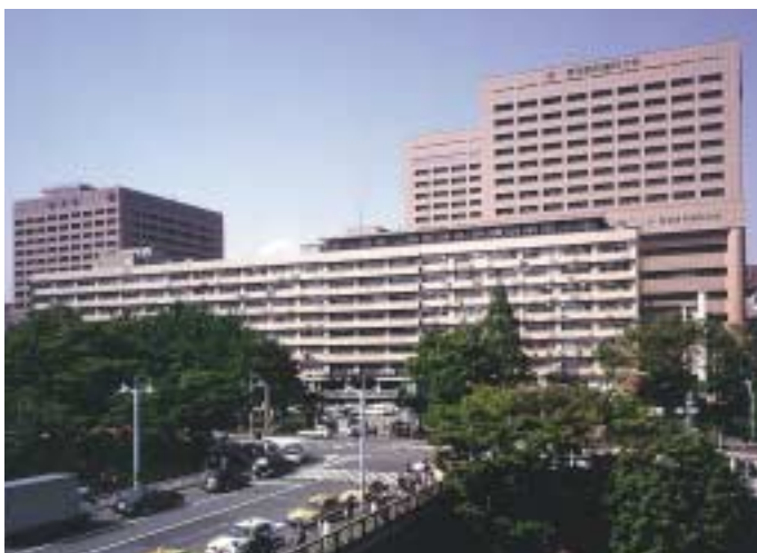
医科棟(診療棟・研究棟)医科新棟 Faculty of Medicine and New Building
