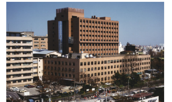
1982(昭和57)年、歯学部附属病棟の歯科新棟が竣工。 In 1982, construction of the new wing of the Dental Hospital was completed, and it is seen in the photo above as the tall building in the center.
